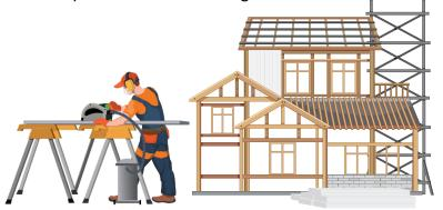
When using a power saw (e.g. track saw, circular saw or drop saw), dusts released must be controlled during work activity.
