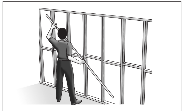
FIGURE 1 FRAME STRAIGHTNESS
